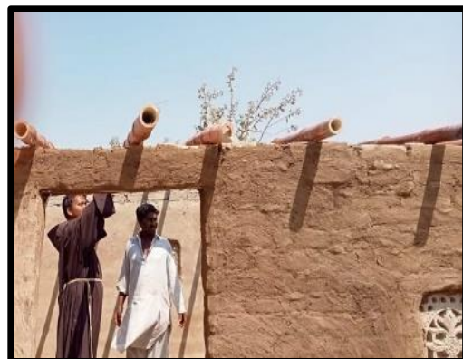
Construction of houses for flood victims Pakistan
